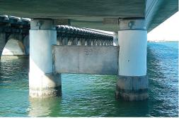
Galvashield DAS Jackets provide protection to pile sections above the tidal zone.
