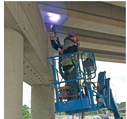
Galvanode® ASZ+ installation
